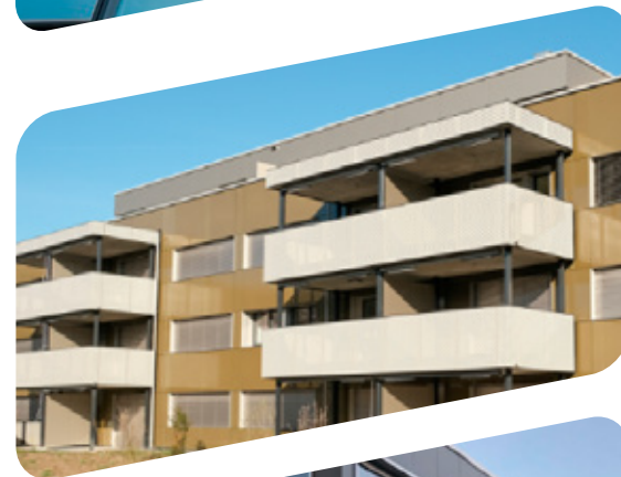
< Münsingen Apartments © Megasol Energie AG
